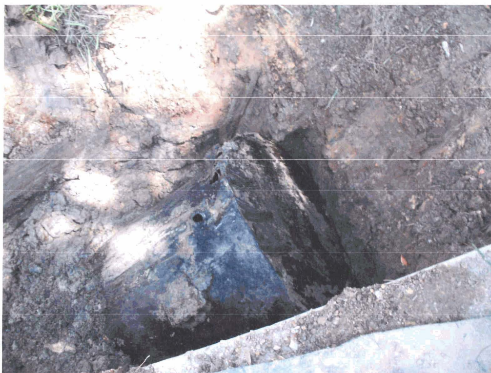
Picture 2: UST 439 Elderberry excavation in progress.
